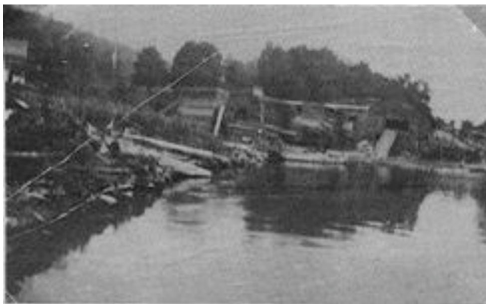
THOMAS CLARK MILL, WINDERMERE: This picture, taken from the lake side of the mouth of the River Dee at Windermere, shows the buildings of the Tom Clark sawmill, with a jack ladder to bring logs up to the saw equipment from where they floated just offshore.
